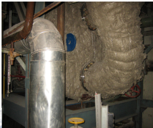
Vahterus PSHE condenser installed at turbine hall #2 at GES-1
