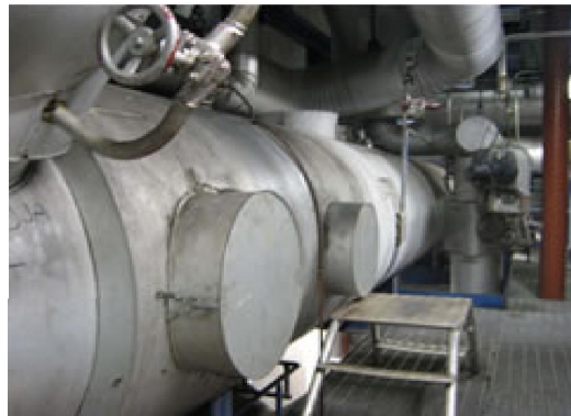
Tubular exchanger LEL2 being dismantled
